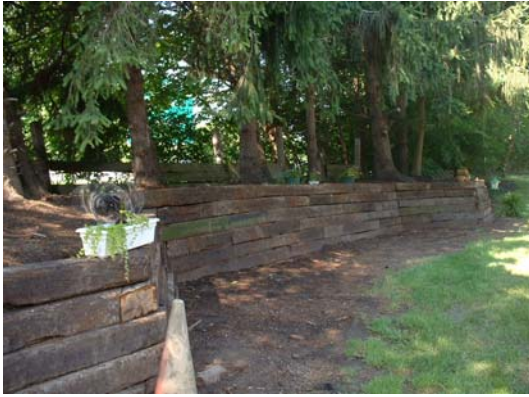
Rebuilt Wall at South Border
