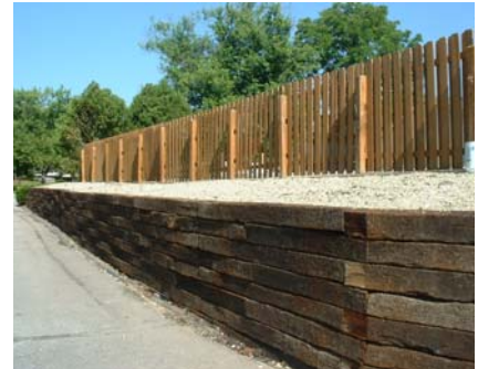
Finished Retainer Wall
