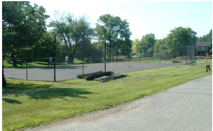
North Court Repaved, Fencing In Progress
