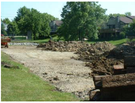
South Court Finally Removed! Fill dirt will be covered with topsoil and seeded with grass.
